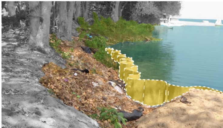
Edges treated with sheet piling to prevent erosion
